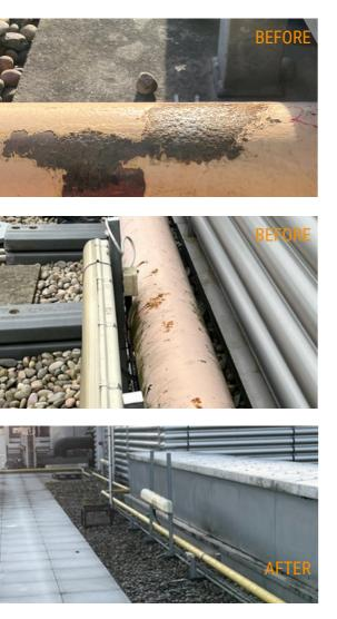
After being exposed to the brutal North Sea weather conditions for 13 years, the natural gas pipework on the roof of Union Square Shopping Centre in Aberdeen, UK was showing signs of deterioration in condition due to corrosion.
