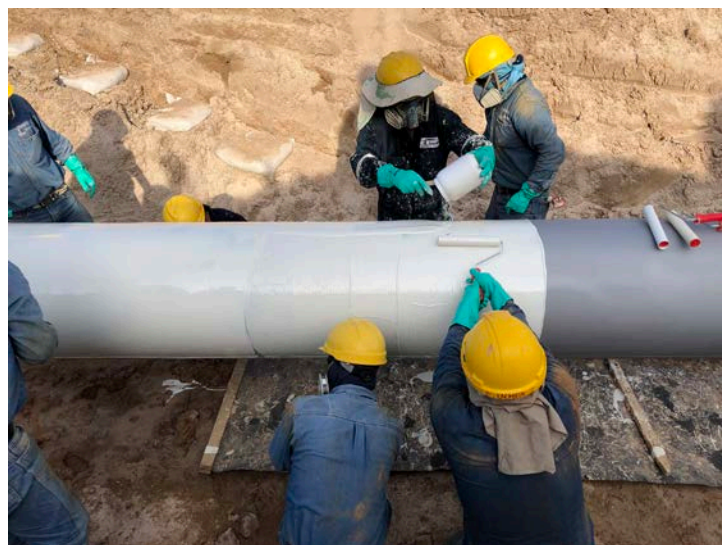
Figure 5. Canusa HBE FLX being applied.
