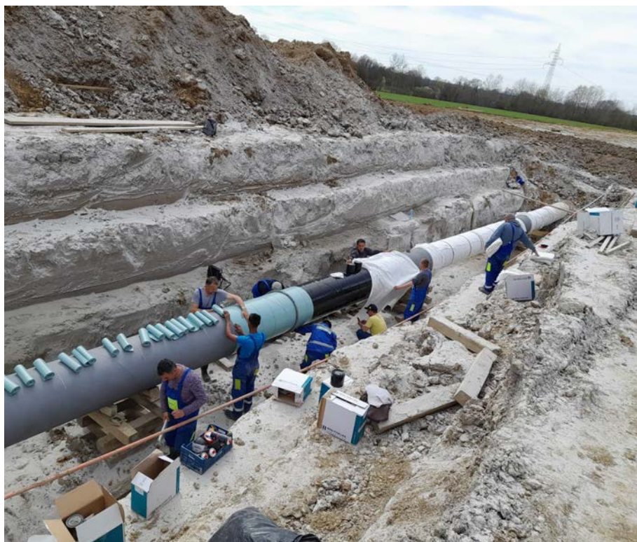
Figure 3. STOPAQ complete protection system for underground installations.
